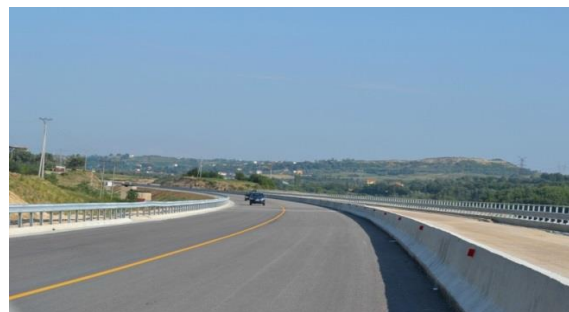
Figure 21: Tirane-Elbasan Road Project, Albania
